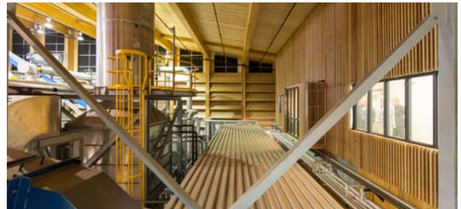
Photos: McFarland Marceau Architects
